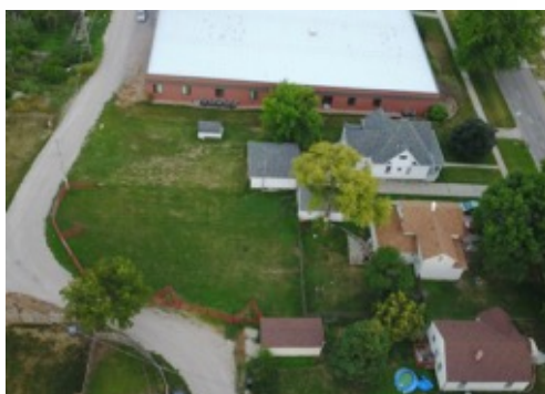
Three lots North of school (seen above) will be home to the new playground
